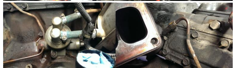
Cut Blue hoses for removal
